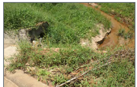
A Troy citizen overlooks a drainage ditch that is eroding her yard as well as the area's streets and drainage structures.
